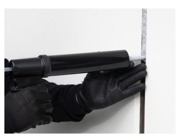
Apply the sealant at a steady pace and in sufficient volume to fill the joint. Make sure the sealant makes contact to both adhesion surfaces.
