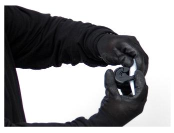
Cut the cartridge nozzle at a 30 degree angle and at the width that corresponds to the size of the joint.
